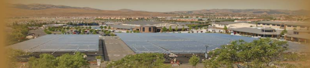
San Ramon Unified School District Solar, Contra Costa County
